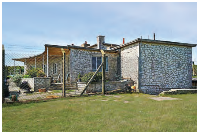
The flat-roofed guard house at Portland was one of the few whose design was modified to incorporate local building materials
